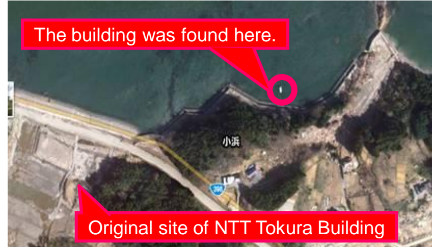
Satellite photo of Tokura Building
