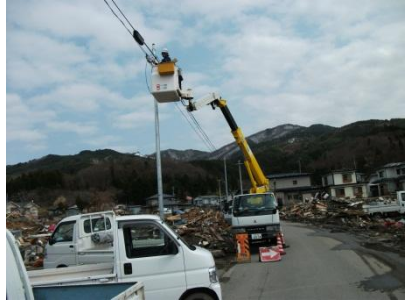
[Step 4] Connections of aerial cables
